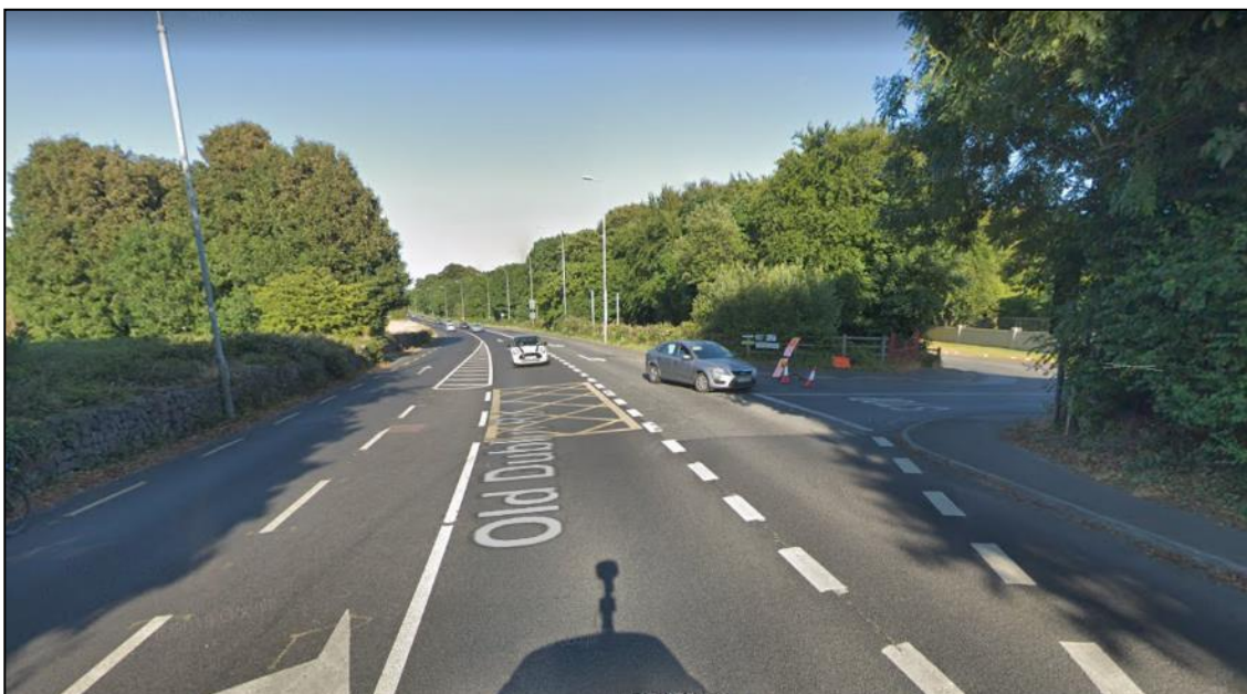
Figure 11.2: Existing Junction (Looking Eastward)
